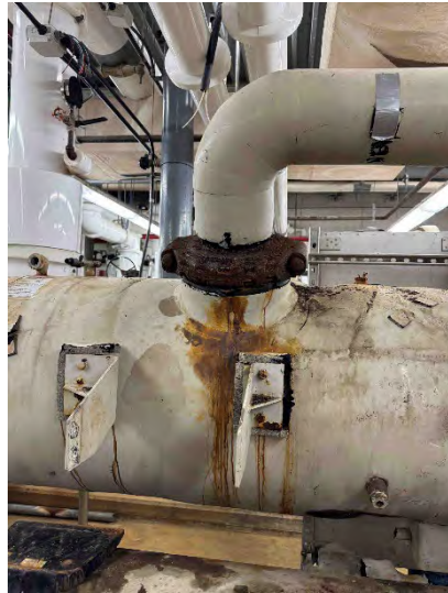
Side View Insulation Around Shell
