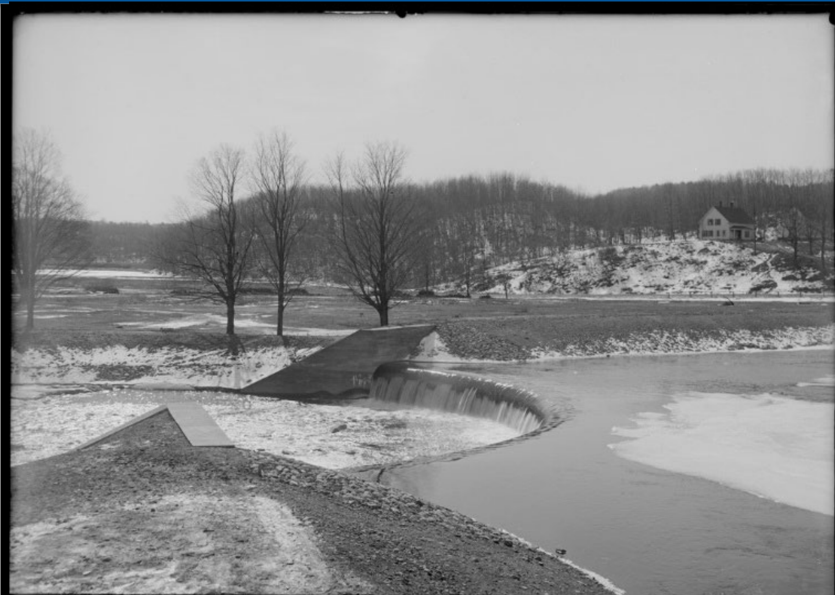
WACHUSETT RES. OAKDALE, CONCRETE DAM ON QUINEPOXET RIVER. FEB. 23, 1906.
