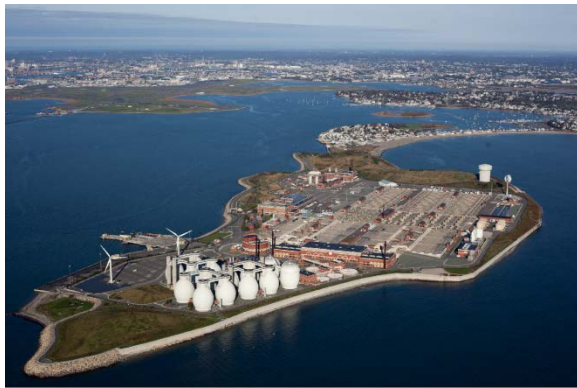
Fig. 1. Deer Island wastewater treatment facility at the mouth of Boston Harbor
