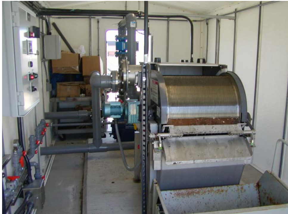
Figure 6-1. Effluent floatables sampler at the Deer Island Treatment Plant.
