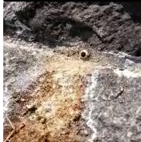
After weep hole cleaning
