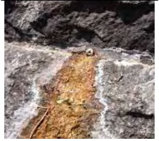
After weep hole cleaning
